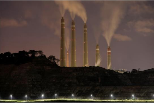
Smoke and steam billows from the coal-fired power plant owned by Indonesia Power, next to an area for Java 9 and 10 Coal-Fired Steam Power Plant Project in Surabaya, Banten province, Indonesia, July 11, 2020. Picture taken July 11, 2020. REUTERS/Willy Kurniawan
